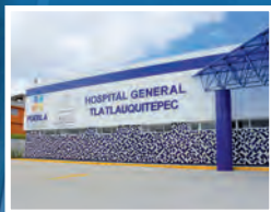
• Hospital General de Tlatlauquitepec
