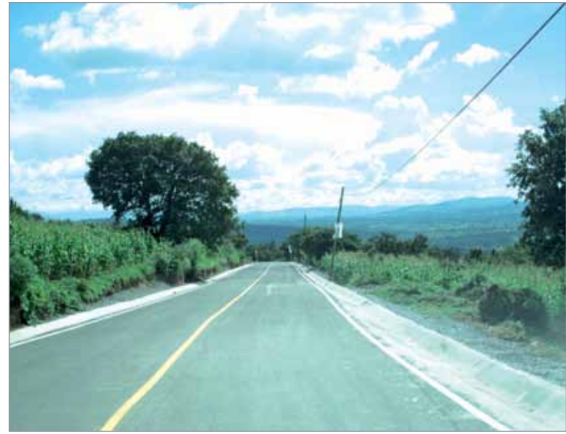
Mayor infraestructura carretera
